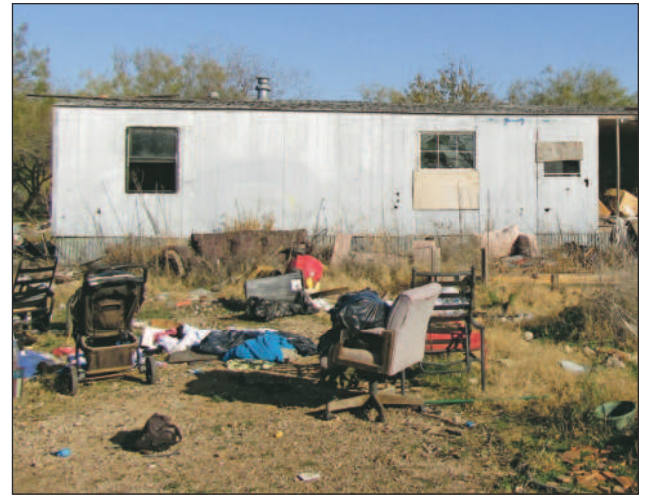
A property at 1208 W. 3rd that was one of six discussed by the Breckenridge City Commission which were determined to be dangerous.
