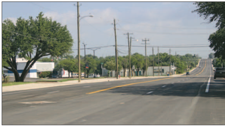
Five years in the making, the US 183 North construction project was fully completed Monday, June 2 and all four lanes -- two northbound and two southbound -- are officially back open to traffic.
